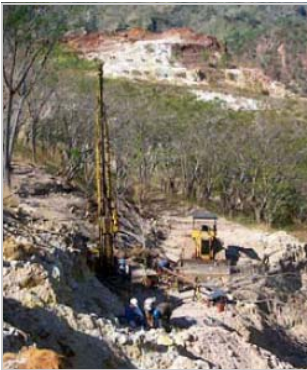
Drill rig on site at Wetar Island
